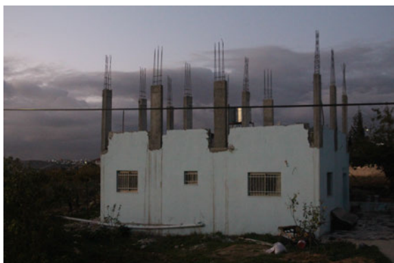
Under Construction , 60cmx40cm, Bil'in 2011.
